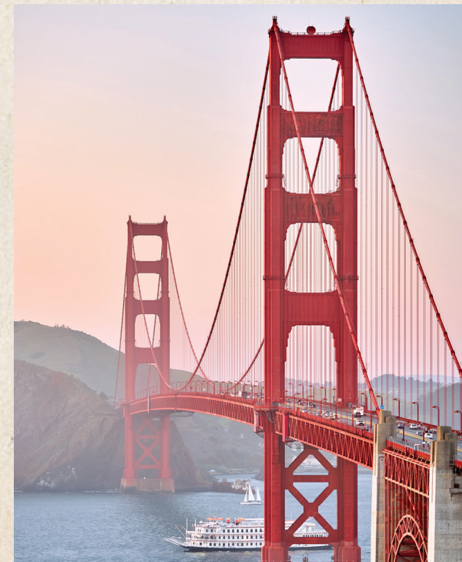
Golden Gate Bridge, San Francisco, CA
